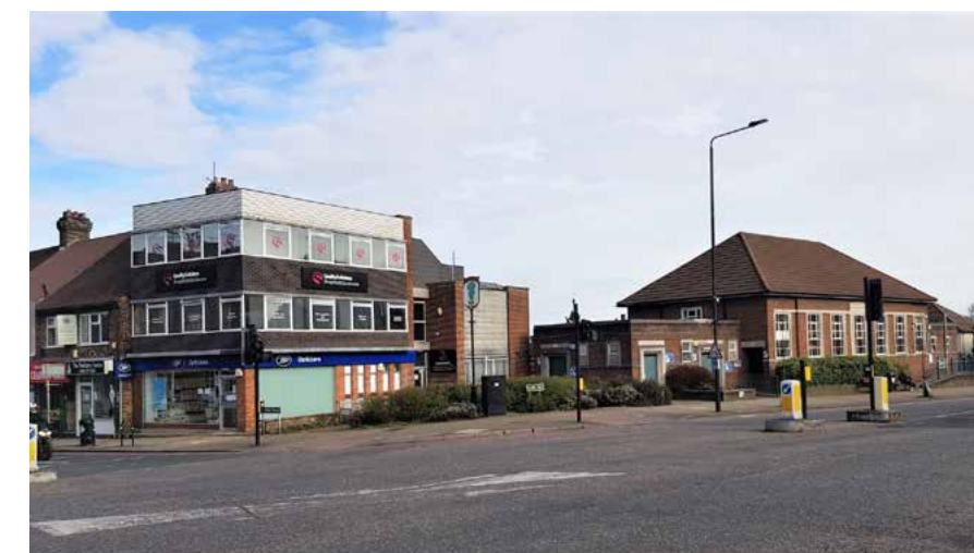
Exposed 1980ies building flanking open plot to library
