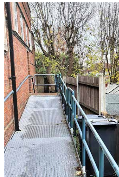
Existing fire escape retained
