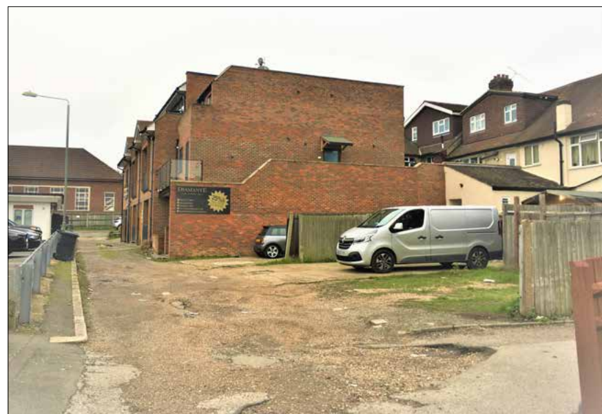
Condition of access road and link to Station Road
